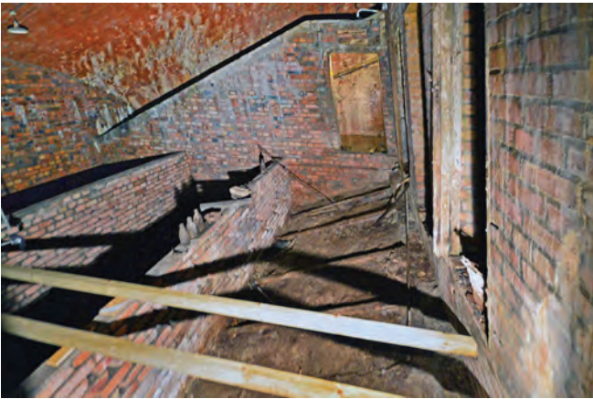
Sections used as offices and for barrage balloon repair
